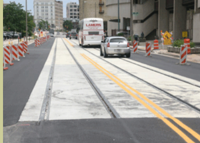
Newly laid section of rubber-booted T-rail track!
